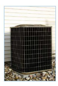
Check your central air conditioner's refrigerant charge and adjust it if necessary to make sure it meets manufacturer specifications. Too much or too little refrigerant charge can damage the compressor, reducing the life of your equipment and increasing costs.
